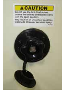
Tank Flush Inlet
